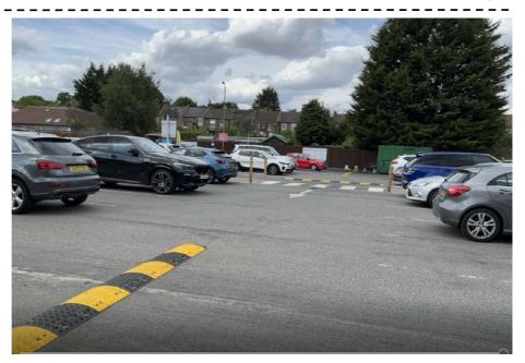
These humps are not sinusoidal in profile which is recommended to minimise discomfort but simple rubber/plastic ones screwed onto the surface. Cheap and nasty in reality.
